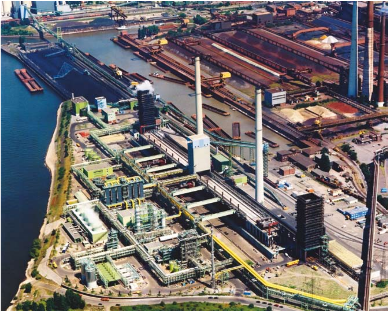
Overview of coke making facility and gas cleaning plant, Germany.
